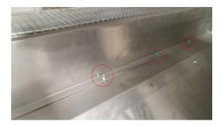
Prior to starting unit back up, Ansul System must be primed, otherwise links will break straightaway
