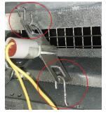
7. Once ETL is installed, use the slipjoint plyers to push hooks closed
